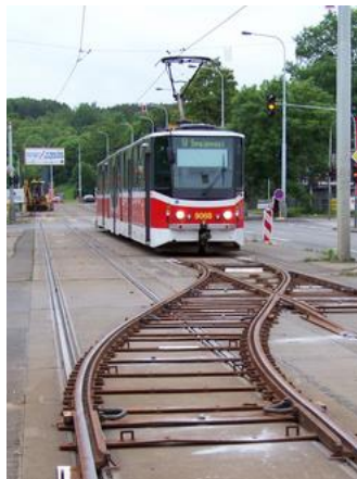
Figure 2: The temporary turning loop [13]
